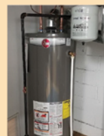
gas & oil water heaters
